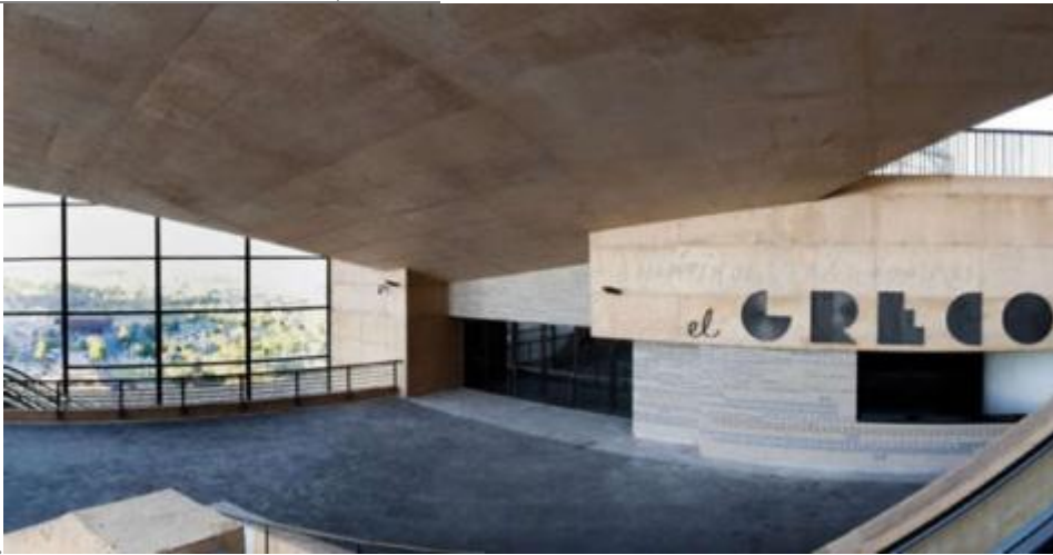
Miradero”. The natural conditions of the site –the topography- allows for the parking lot to be designed with entrances and exits from the lower level, while the congress centre accesses are made available from the historic city centre
