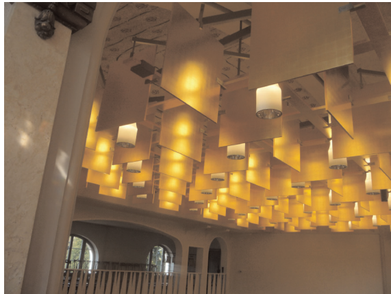
Figure 5. Photo of diffuser after the refurbishment
