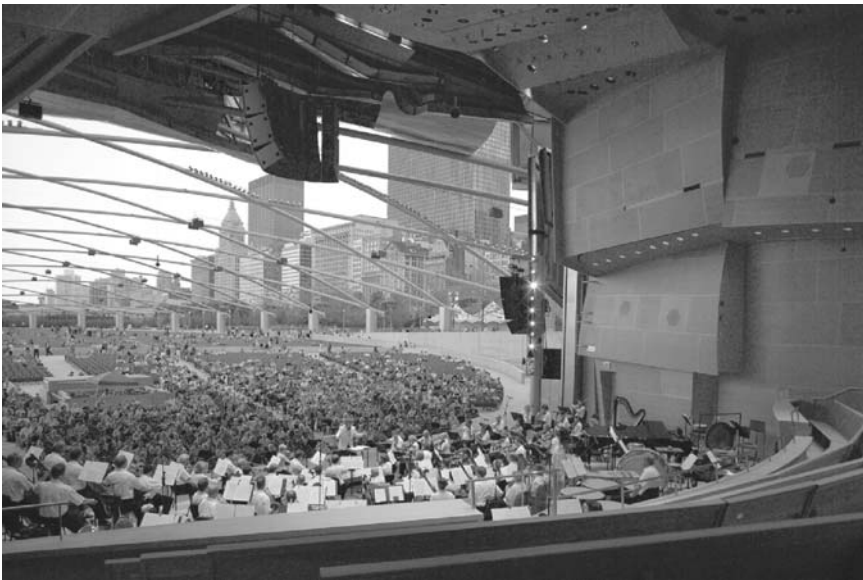
FIGURE 11.20. View from the stage of the Pritzker Pavilion. The trellis overhead of the audience contains a distributed loudspeaker system.
