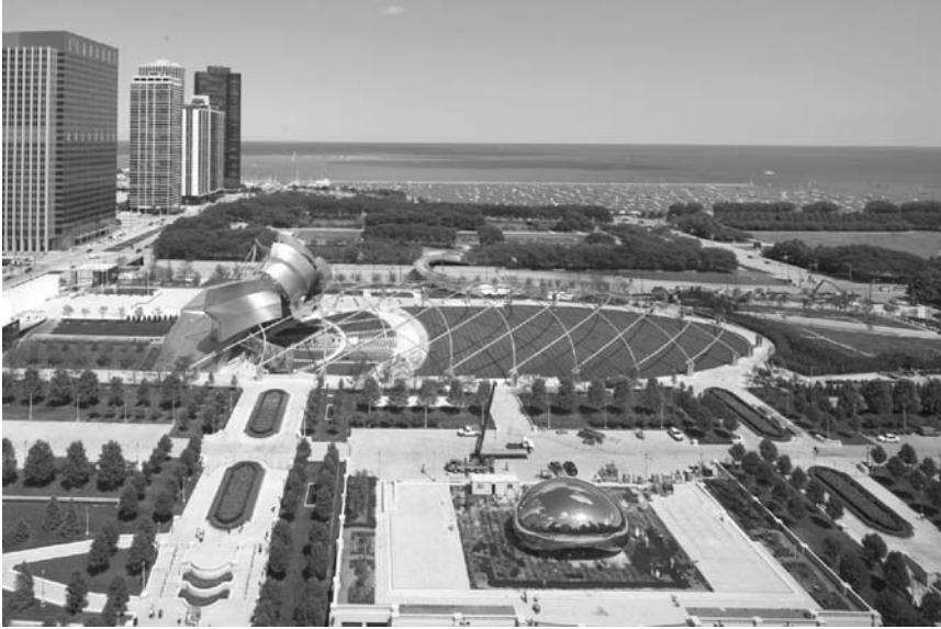
FIGURE 11.18. The Jay Pritzker Pavilion in Chicago. The radical design also features a trellis system from which loudspeakers are suspended. (Courtesy of TALASKE, graphics by DOXA.)
