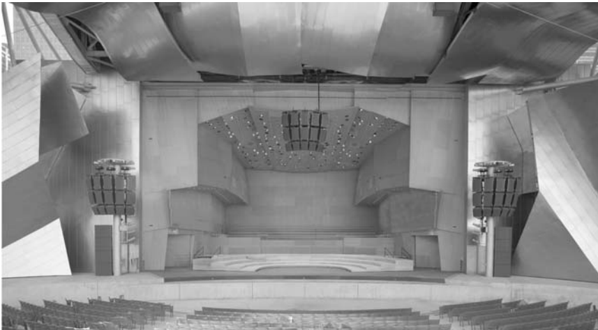
FIGURE 11.19. The stage of the Pritzker Pavilion can accommodate an orchestra of more than 100 members plus a 150-member chorus. (Photograph by Richard H. Talaske.)
